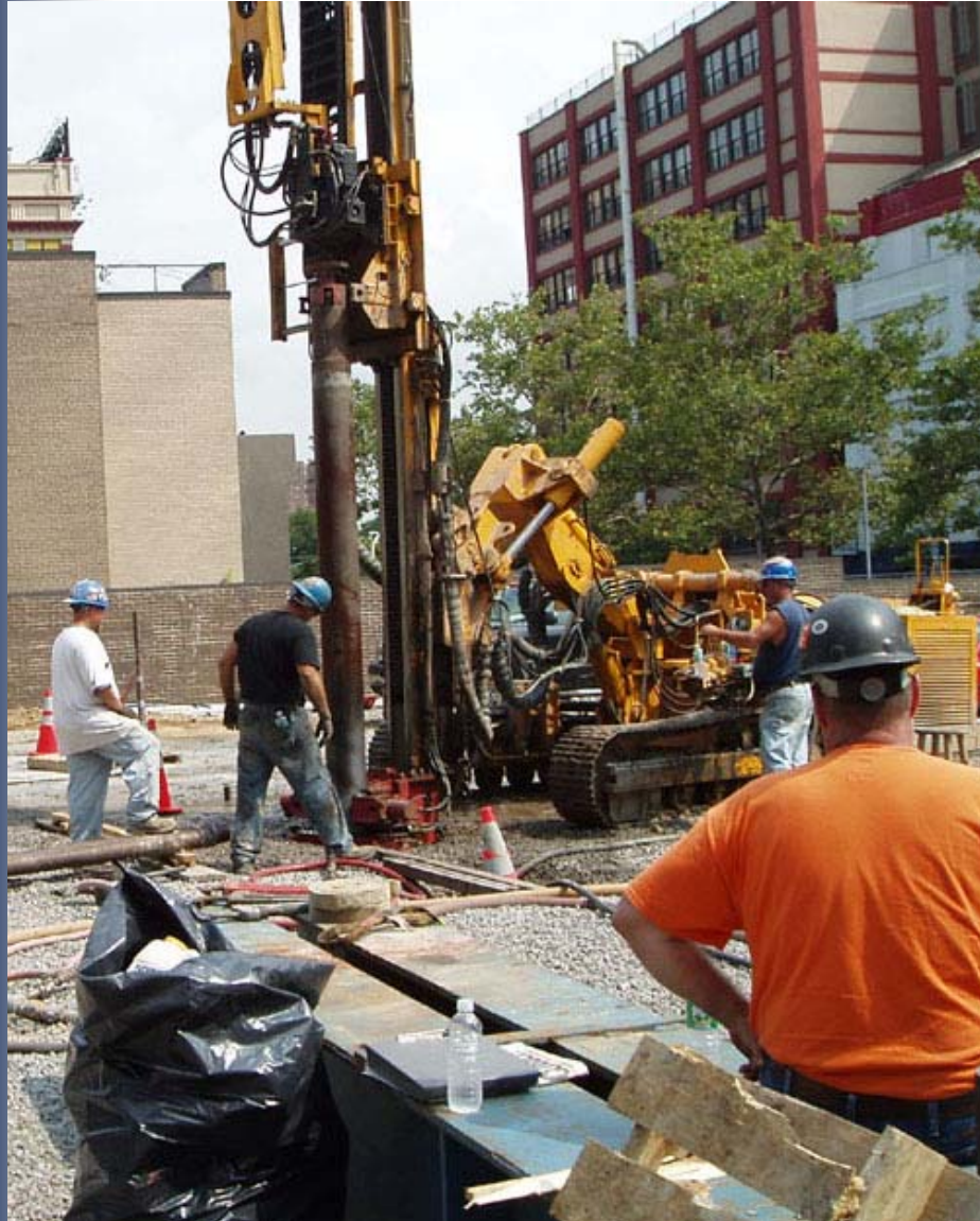
Left - Installation of 273 mm test element (pile) Top – Buried old foundation wall and obstructions
